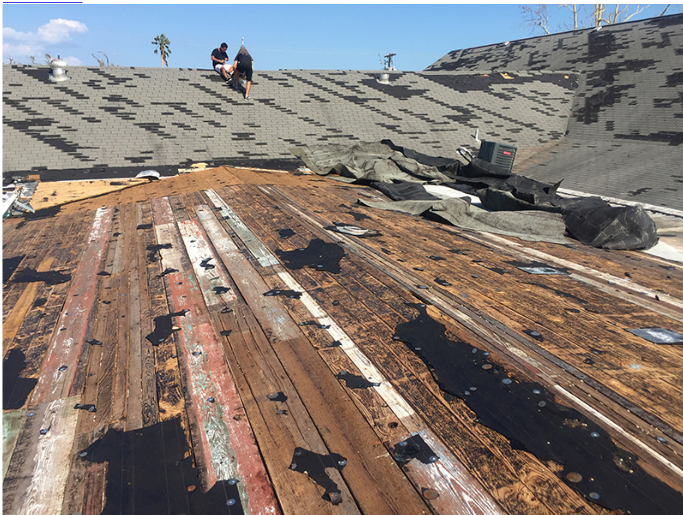
Damage to the roof of the Rockport Assembly of God Church after Hurricane Harvey in Rockport, Texas. (Courtesy of Becket Law Firm)
