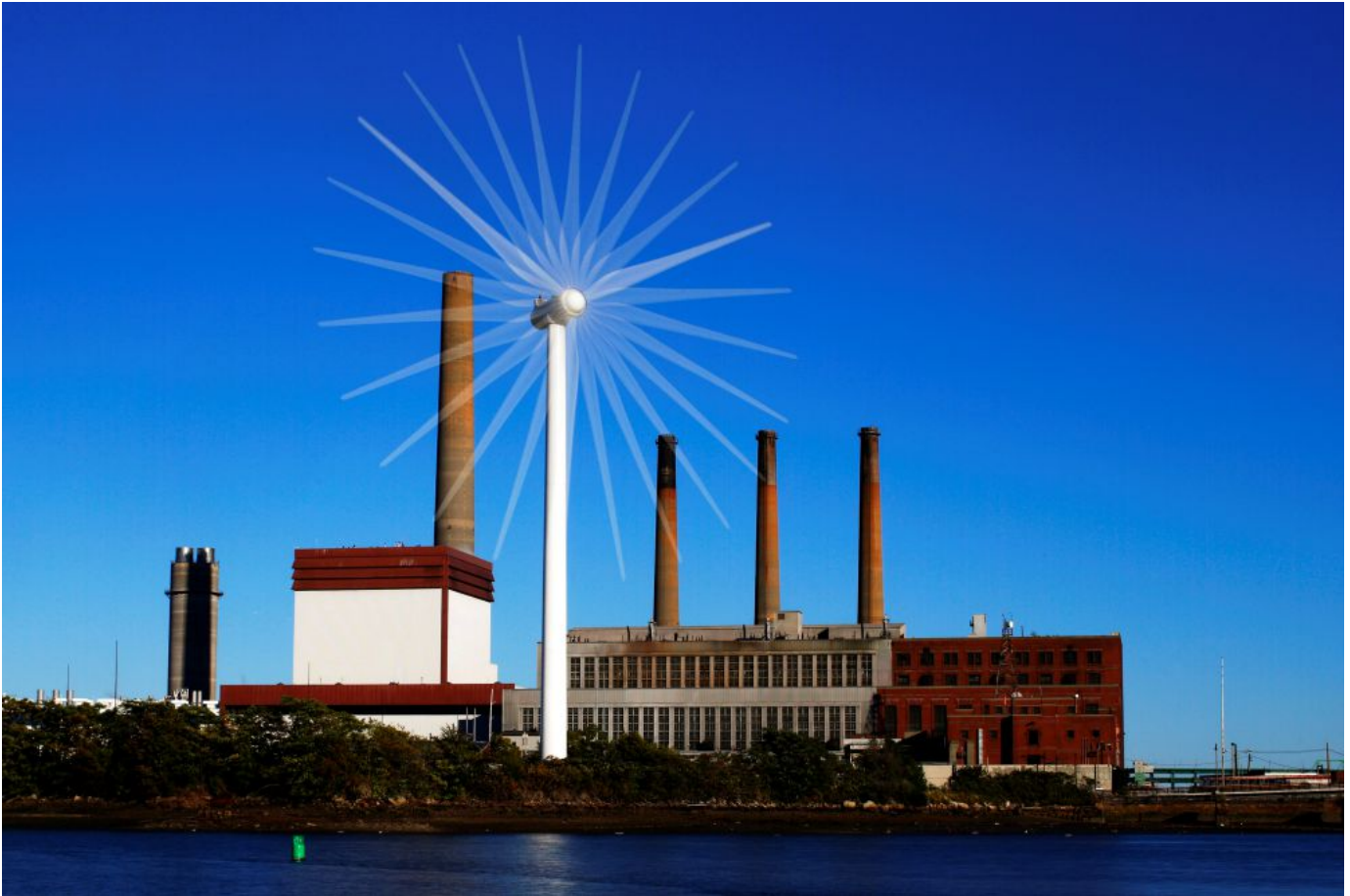
Wind turbine in front of a fossil fuel power plant in Charlestown, Massachusetts, 2013 (CNS/Reuters/Brian Snyder)
