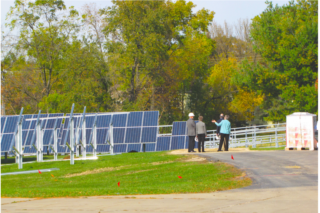
Touring the solar panel array in 2014, when they were about one year old on the property of the Franciscan Sisters of Rochester, Minnesota (Franciscan Sisters of Rochester, Minnesota)
