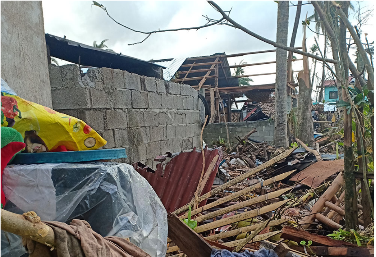
Debris from houses and fallen trees in San Francisco, Southern Leyte. (Courtesy of the Religious Sisters of Mercy)
