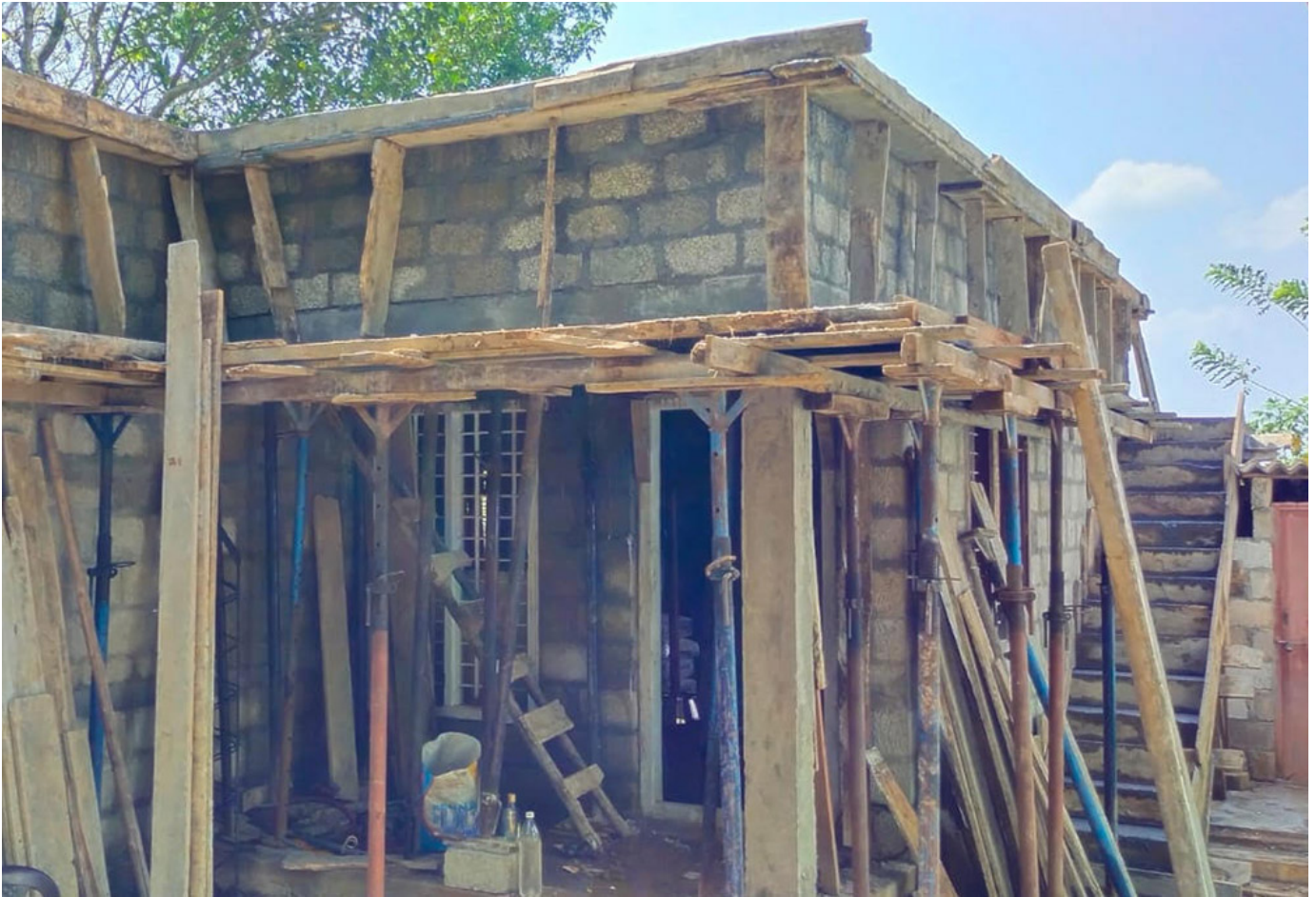
The walls of the new house under construction (Courtesy of Rose Cherian Vachaparampil)
