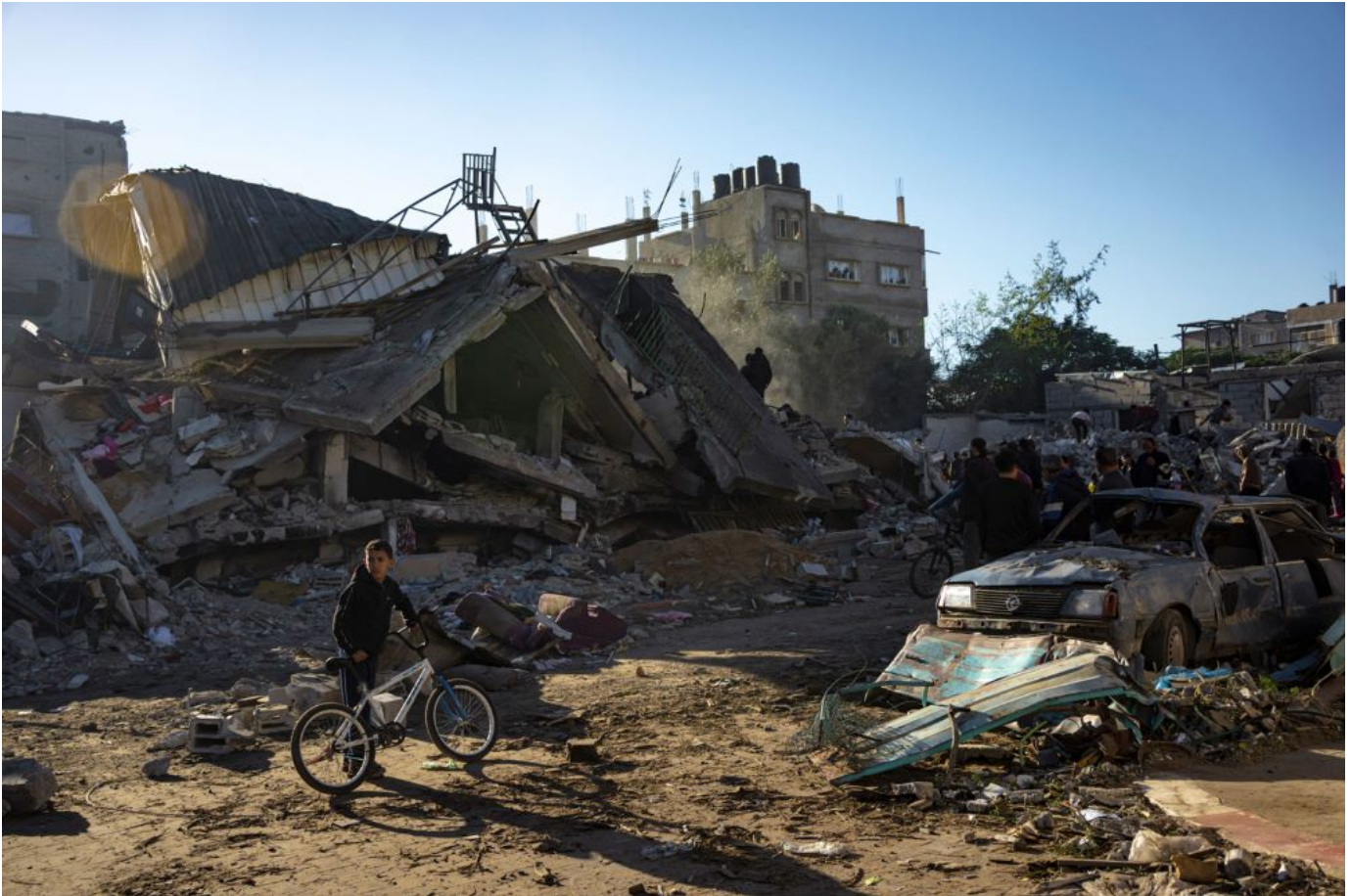
Palestinians search for bodies and survivors in the rubble of a residential building destroyed in an Israeli airstrike, in Rafah, southern Gaza Strip, on Dec. 15. (AP/Fatima Shbair)
