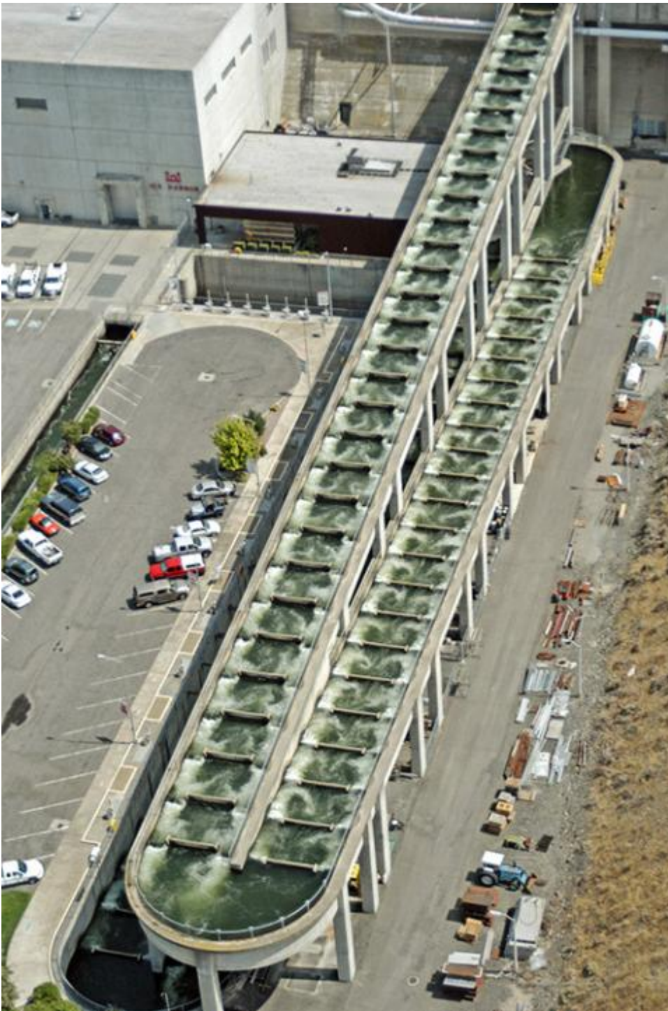
A fish ladder at Ice Harbor Dam on the lower Snake River in Washington (Wikimedia Commons/Bonneville Power)
