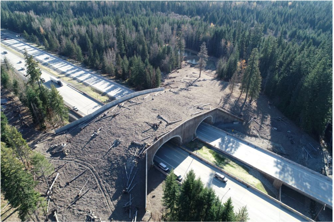
A land bridge crossing for wildlife over Interstate 90 is seen near Snoqualmie Pass, Wash., Oct. 30, 2019. (OSV News/Washington State Department of Transportation/Handout via Reuters)
