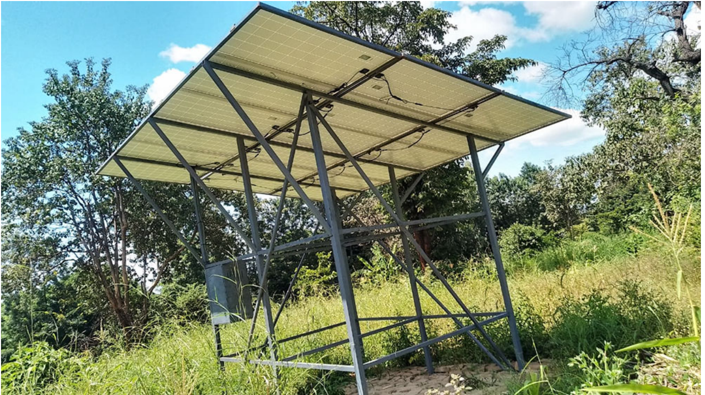
Solar panels power the borehole in Mashuru Community in Kajiado County, Kenya. (Courtesy of Beatrice Kamau)
