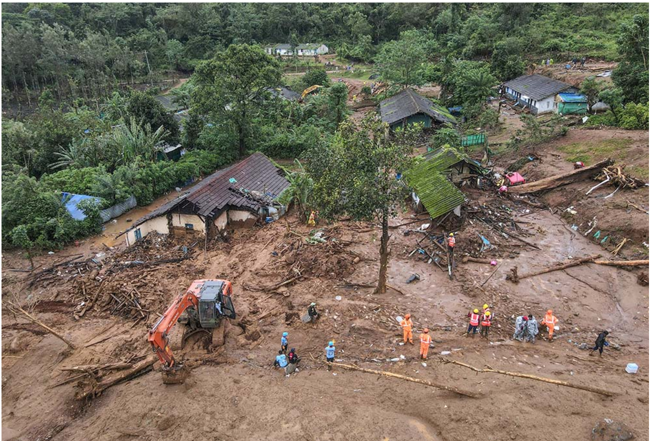
A drone view shows destroyed homes in the southern state of Kerala, India, Aug. 1, following multiple landslides in the hills in Wayanad district. (OSV News/Reuters/Francis Mascarenhas)
