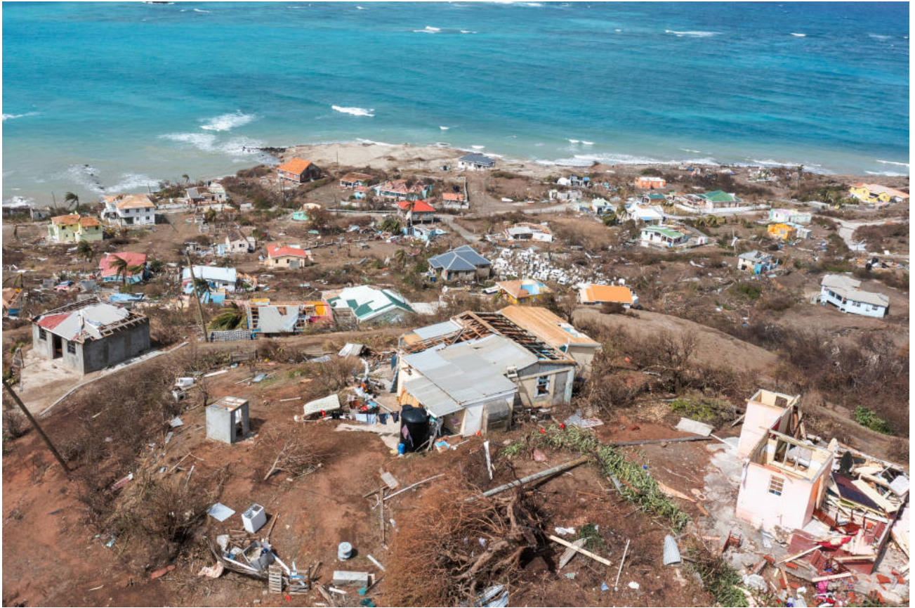
Scattered debris and houses with missing roofs are seen in a drone photograph July 2, 2024, after Hurricane Beryl passed the island of Petite Martinique, Grenada. (OSV News photo/Arthur Daniel, Reuters)
