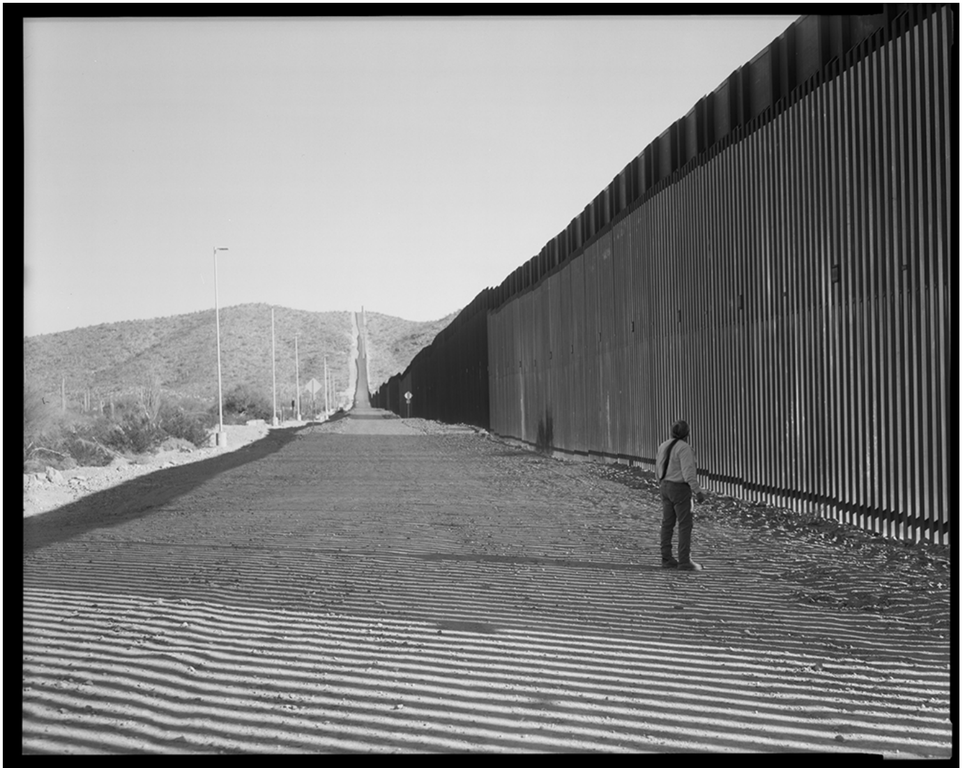
Samuel Fayuant stands before Monument Hill in the Organ Pipe Cactus National Monument, a sacred place where O'odham ancestors have been buried. The wall built during the Donald Trump presidency runs through this sacred ground. (Lisa Elmaleh)
